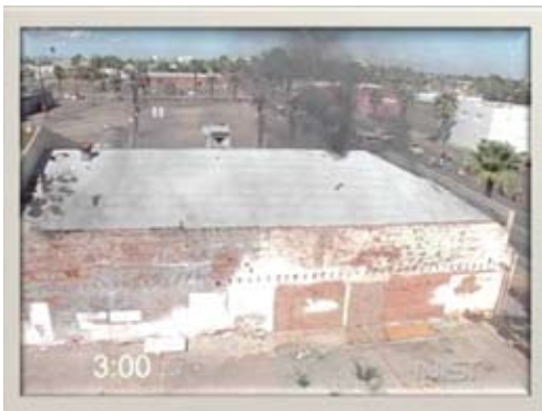
Three minutes after ignition, there is plenty of fuel and plenty of oxygen so the temperature climbed steadily toward flashover.
