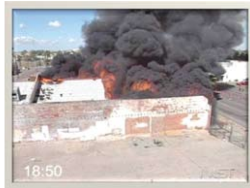
Eighteen minutes after ignition, 10 minutes after the front door was opened, a large area of the roof has collapsed. So much for the so-called "20-minute rule."
